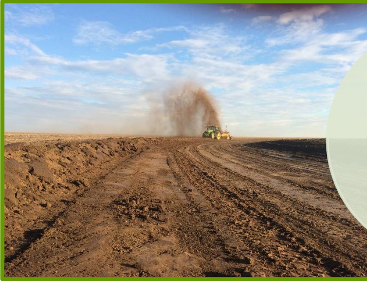
Waterway Repair Addington Farm, McLean County
