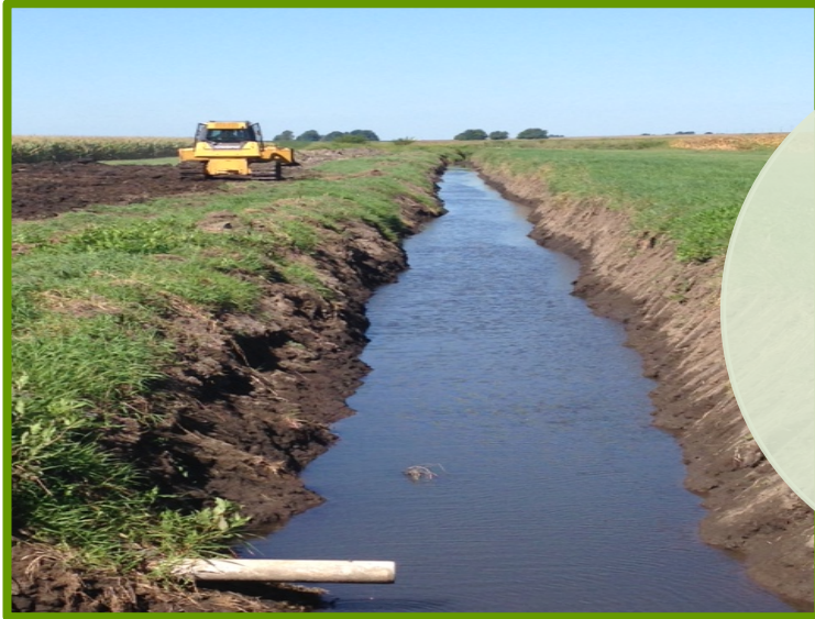
Drainage Ditch Maintenance Hunter Farm, Sangamon County
