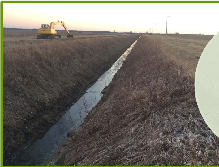
Drainage Ditch Maintenance, Allerton Farms, Piatt County
